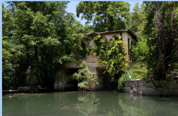
Brackenridge Pump House #1, 1877
