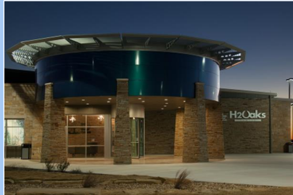
Desalination, 2016 Reverse Osmosis
