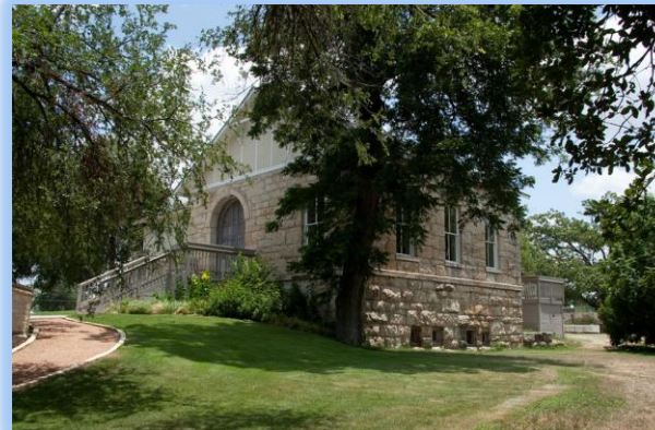
Brackenridge Pump House #2, 1885 The Borglum House
